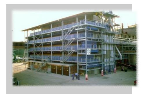
For bigger capacities, several dryers can be installed one on top of the other to save floor space
