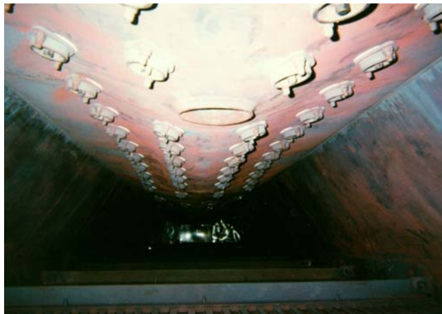
Figure C-2 - Deaerator Spray Nozzles And Trays
