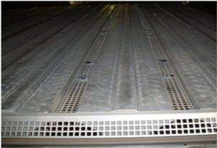
After- new bars and return screens
