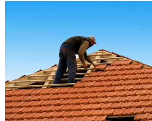
Roof Tiles and Siding
