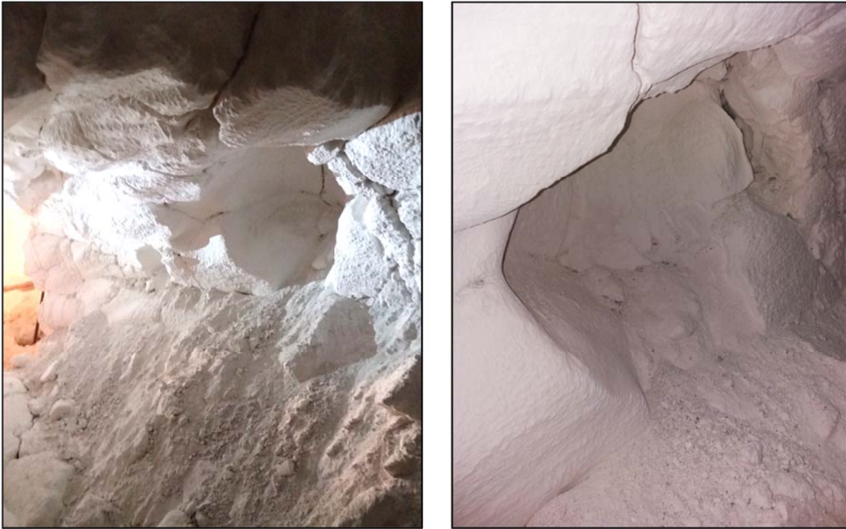
Figure 8. Holes formed in rings as a result of liquid CO 2 blasts.
