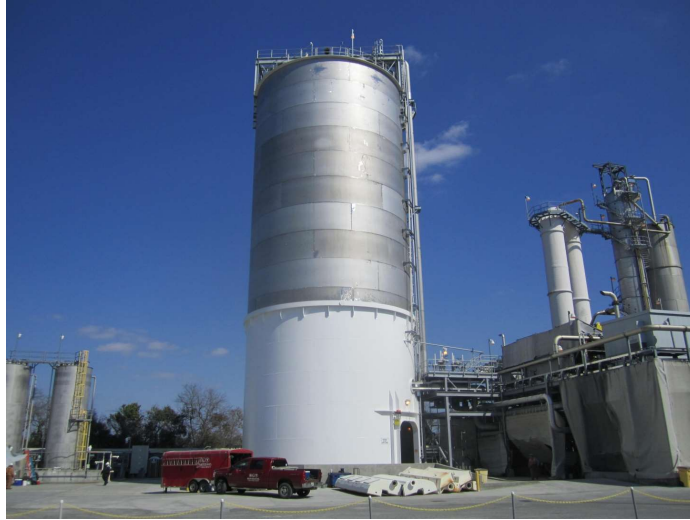
Figure 12. 2205 duplex stainless steel pre-breach storage tank.
