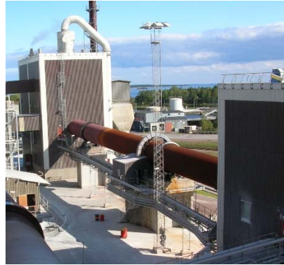
Figure 55. Lime kiln no 2, in which the experimental trials were carried out.
