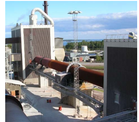
Mönsterås Lime Kiln No 2 275 tonnes of lime per day, dried bark powder and bio-oil
